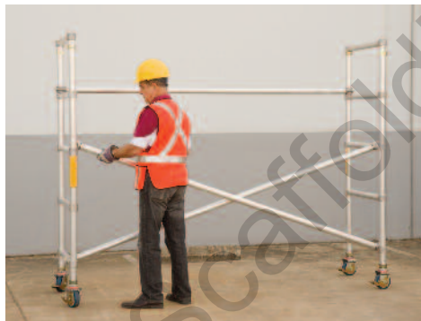
2. Snap long braces (diagonal) in desired position. Horizontal brace must be above or below intersection of diagonal braces.
