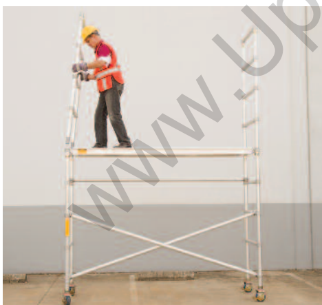
1. Lock all casters. Adjust legs to level platform. Insert extension frames. Interlock all frames by moving interlock clips from parking holes up to locking holes (see page 3).
