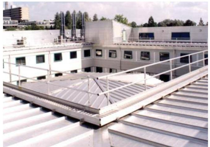
Access over profiled roof to air conditioning plant - Bath University.
