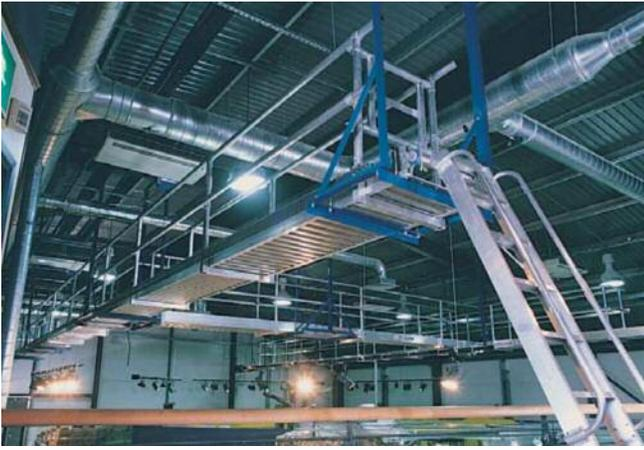
The permanent installation of a suspended Spandek walkway in the Royal Signals Museum provides access to roof work areas such as air conditioning without closing exhibition to the public.
