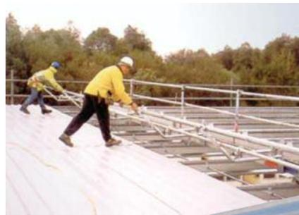
Lightweight trailing edge protection frame offers safe and easy manoeuvrability.
